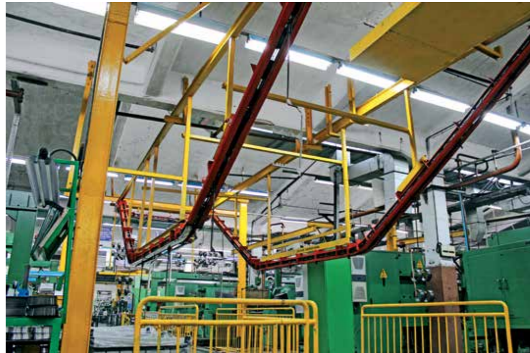
↑ Conveyors take the parts of railway bearings for phosphating process
