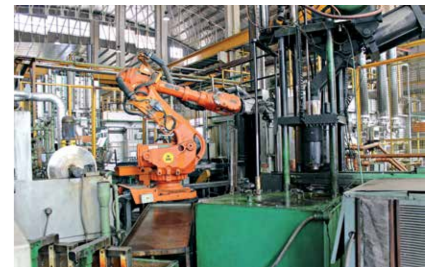
➔ Robot deployed in heat treatment process
